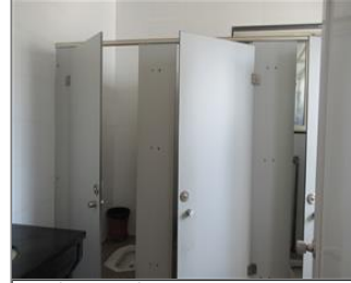
Photo of the sanitary facilities Toilets.JPG
