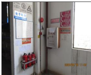
Photo of fire safety equipment Extinguishers hydrant and fire alarm.JPG
