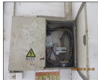
Photo of non-conformity NC-No inner cover for switch box.JPG
