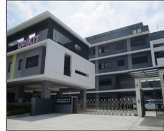
External photo(s) of the production unit(s) Facility outlook.jpg
