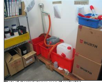
Photo of chemical storage room (if applicable) Chemical containers with 2nd containment and posted MSDS.jpg
