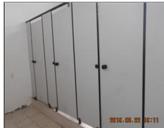
Photo of the sanitary facilities Toilet.JPG
