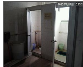
Photo of the sanitary facilities wash room.jpg
