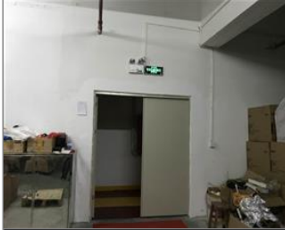
Photo of fire safety equipment Fire exit with emergency light and exit sign.JPG
