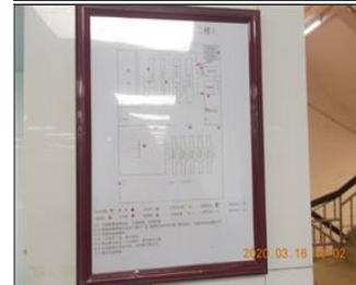
Photo of fire safety equipment Evacuation map.JPG
