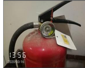
Photo of the inside of the main production hall Pressure of fire extinguisher was adequate.jpg
