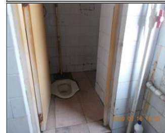
Photo of the sanitary facilities Toilet.JPG
