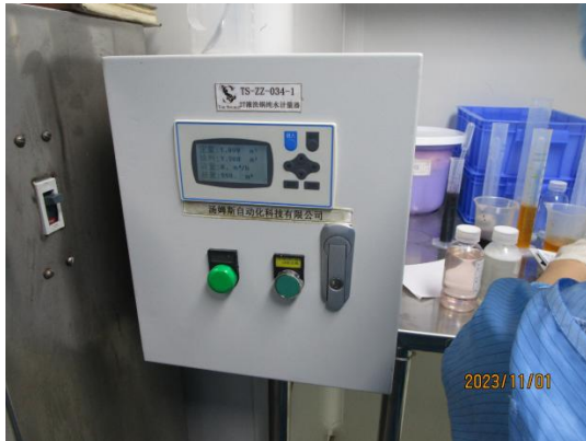
NC Electrical Box not Posted with Warning Sign.JPG
