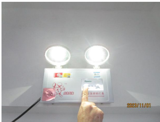
Emergency Lights Testing.JPG
