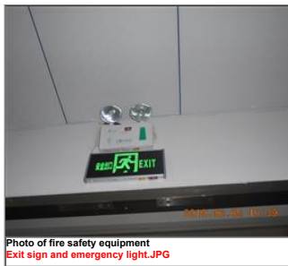
Photo of fire safety equipment Evacuation light.JPG
