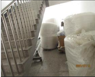
External photo(s) of the production unit(s) NC 7.9 Combustible material stored in stairwell.JPG
