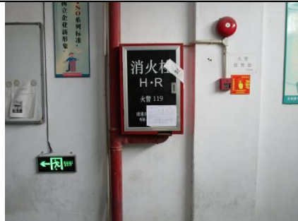
Image 11: Fire hydrants and fire alarms were fully installed.
