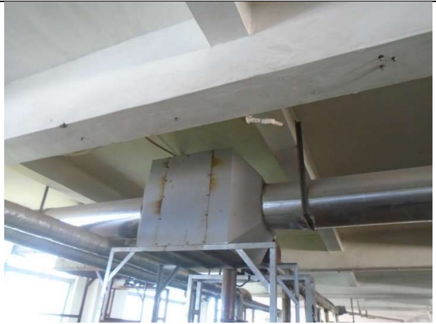
Treatment Facility for Odour from the Decal Firing Production Line #1
