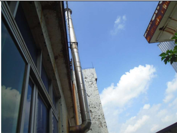
Discharge Outlet for Odour from the Decal Firing Production Line #1
