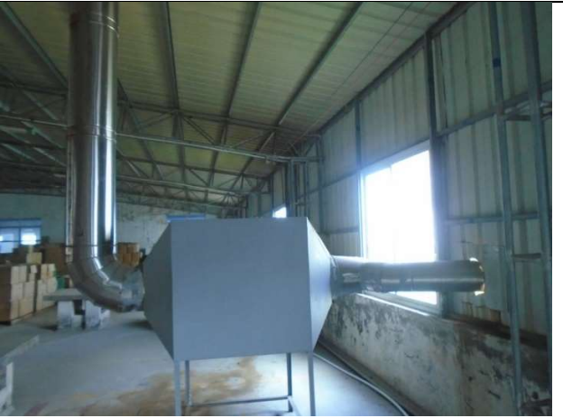
Treatment Facility for Odour from the Decal Firing Production Line #3
