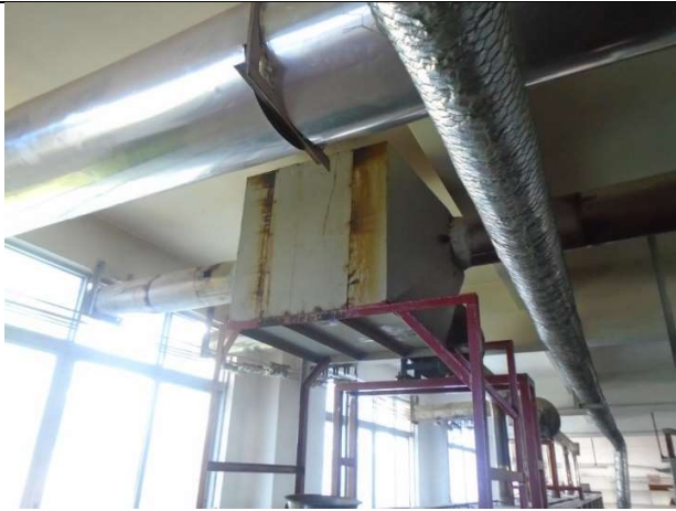
Treatment Facility for Odour from the Decal Firing Production Line #2
