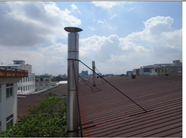
Discharge Outlets for Odour from the Decal Firing Production Lines #2&3
