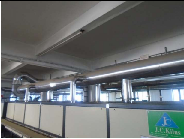
Collection Facility for Odour from the Decal Firing Process
