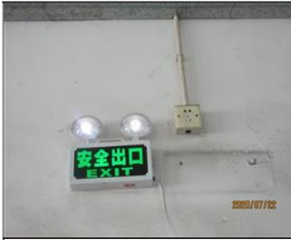
External photo(s) of the production unit(s) Exit sign and emergency light testing.JPG
