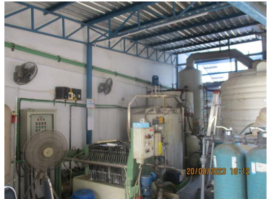
Water Treatment Plant.JPG
