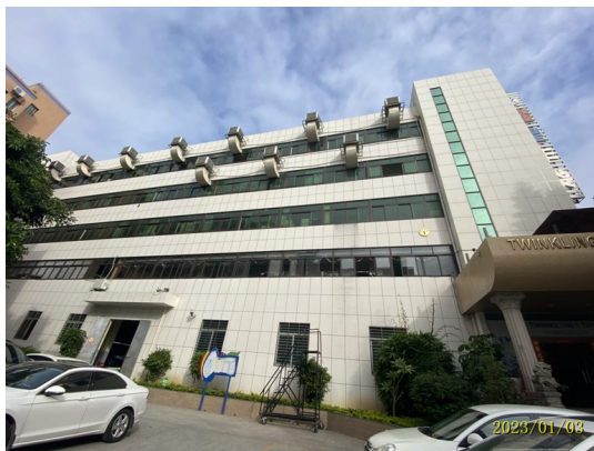
One 5-storey production building.JPG
