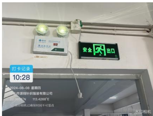
17. Emergency light testing.JPG
