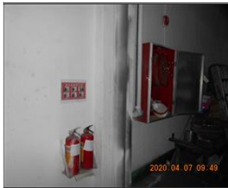
Photo of fire safety equipment Fire extinguishers Fire hydrant and Fire alarm.JPG
