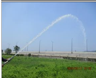
Photo of fire safety equipment Fire hydrant test.JPG
