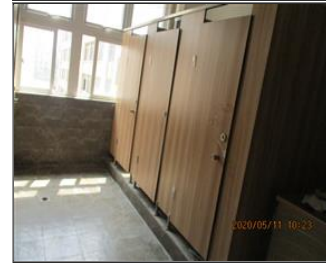
Photo of the sanitary facilities Toilet.JPG
