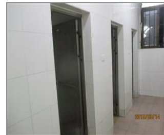
Photo of the sanitary facilities Toilet.JPG
