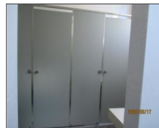
Photo of the sanitary facilities Toilet.JPG
