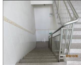
Photo of the inside of the main production hall stair case.JPG
