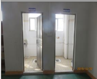
Photo of the sanitary facilities toilets.JPG
