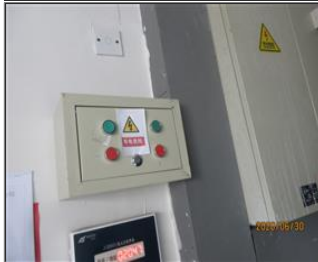
Photo of the inside of the main production hall 9-9 Warning sign.JPG
