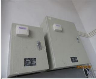
Photo of non-conformity NC - 7.13 No electric shock warning signs were available on electrical distribution box.JPG
