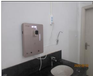
Photo of the sanitary facilities 13-1 Drinking water.JPG
