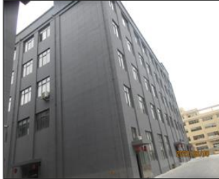
External photo(s) of the production unit(s) 1-2 Factory compound.JPG
