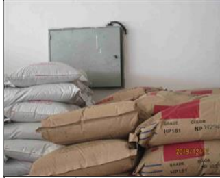
External photo(s) of the production unit(s) 7-9 and 7-13 Without warning sign and Full blocked electric box.jpg
