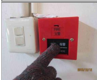
External photo(s) of the production unit(s) Test fire alarm.jpg
