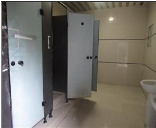
Photo of the sanitary facilities Toilet.JPG
