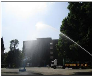
Photo of fire safety equipment Hydrant testing.JPG
