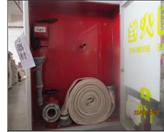
Photo of fire safety equipment Fire hydrant.JPG
