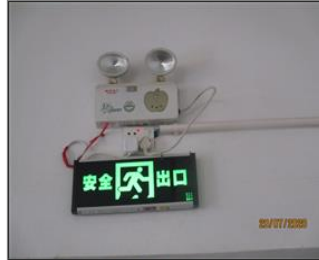
Photo of fire safety equipment Emergency light and safety exit signs.JPG
