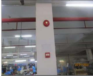
Photo of fire safety equipment Fire alarm.JPG
