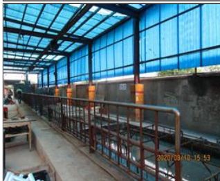
Photo of the inside of the main production hall Pre-treatment process.JPG
