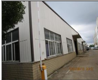
External photo(s) of the production unit(s) Production buildings.JPG
