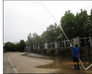
Photo of fire safety equipment Fire hydrant testing was OK.JPG
