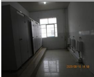
Photo of the sanitary facilities Toilets.JPG
