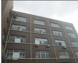
External photo(s) of the production unit(s) Workshop building.JPG
