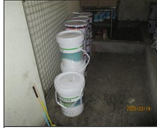
Photo of non-conformity NG 7.7 No secondary container.JPG
