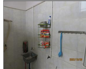
External photo(s) of the production unit(s) sink of toilet.JPG
