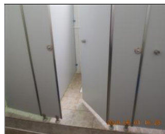
Photo of the sanitary facilities Toilet.JPG
