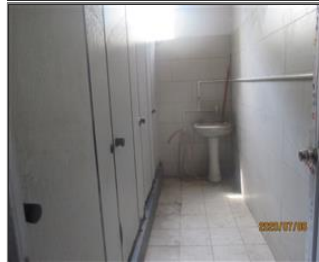
Photo of the sanitary facilities Restroom.JPG
