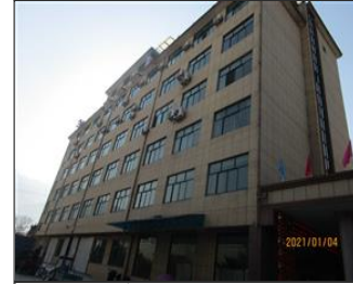
External photo(s) of the production unit(s) 3.Complex building.JPG
